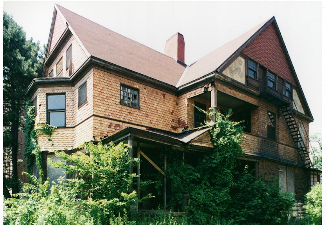
W.R. Allen House, Pittsfield 2006
