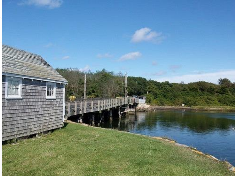
Mitchell River Bridge, Chatham MER
