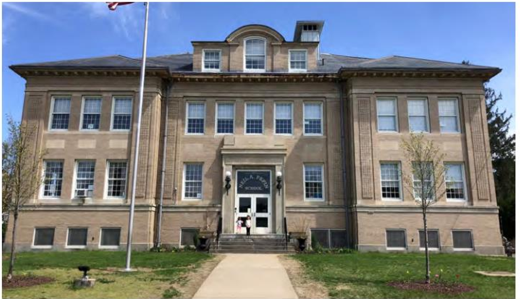
Image 25: The exterior facade of Pepin Elementary School.
