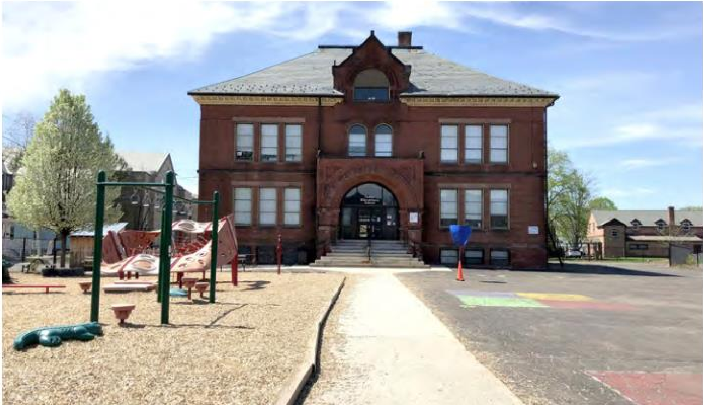
Image 22: Center Elementary School Yard.
